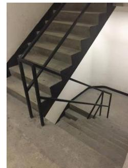
Fig. 7. Stairs only accommodate space for one occupant at a time to descend.
